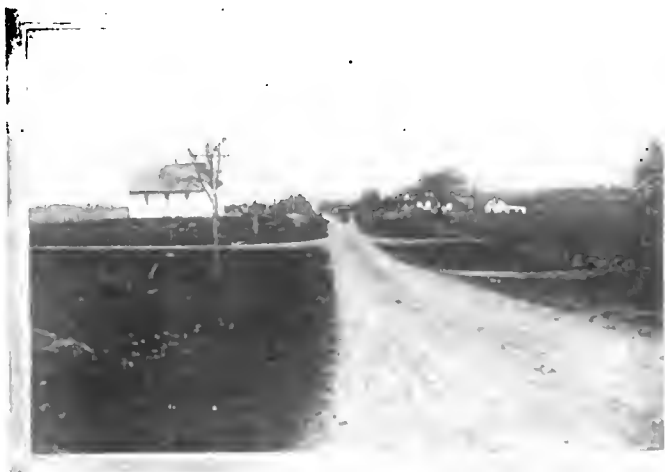
FORTY MILES OUT FROM SOUTH BEND, INDIANA.
